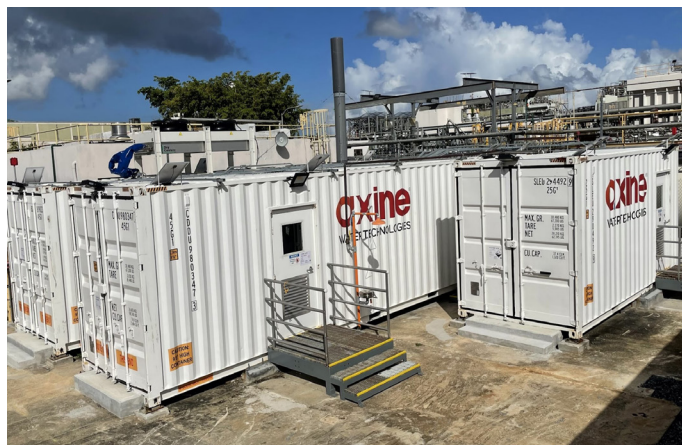
Axine's on-site system installation
